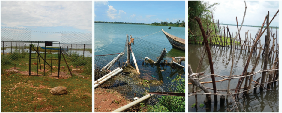
Figure 2. Examples of crocodile exclusion enclosures: two dysfunctional and one functional. From left to right: a dry enclosure due to a drop in the water level in Lwanika followed by an enclosure that was destroyed by strong winds in Daguzi, and lastly a locally made enclosure in Mubaku, MFCA.
